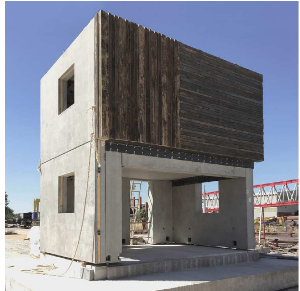
Figure 2 Demo building in Madrid
